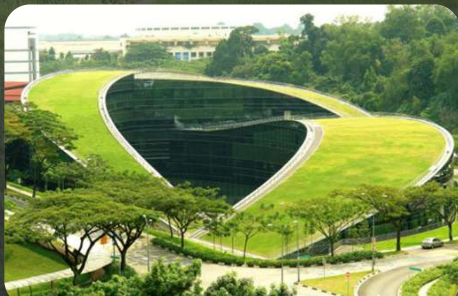
The incredible green roof at the School of Art, Design and Media at Nanyang Technical University in Singapore [18]
