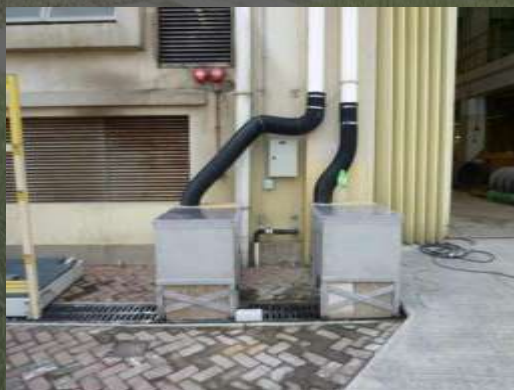
V-notch weir chamber (runoff measurement)
