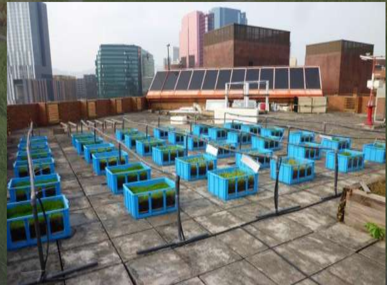
Actual setup on the roof of PolyU, building-P 8 October 2012
